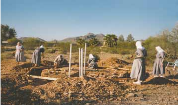
Sisters assisting as foundations are laid
